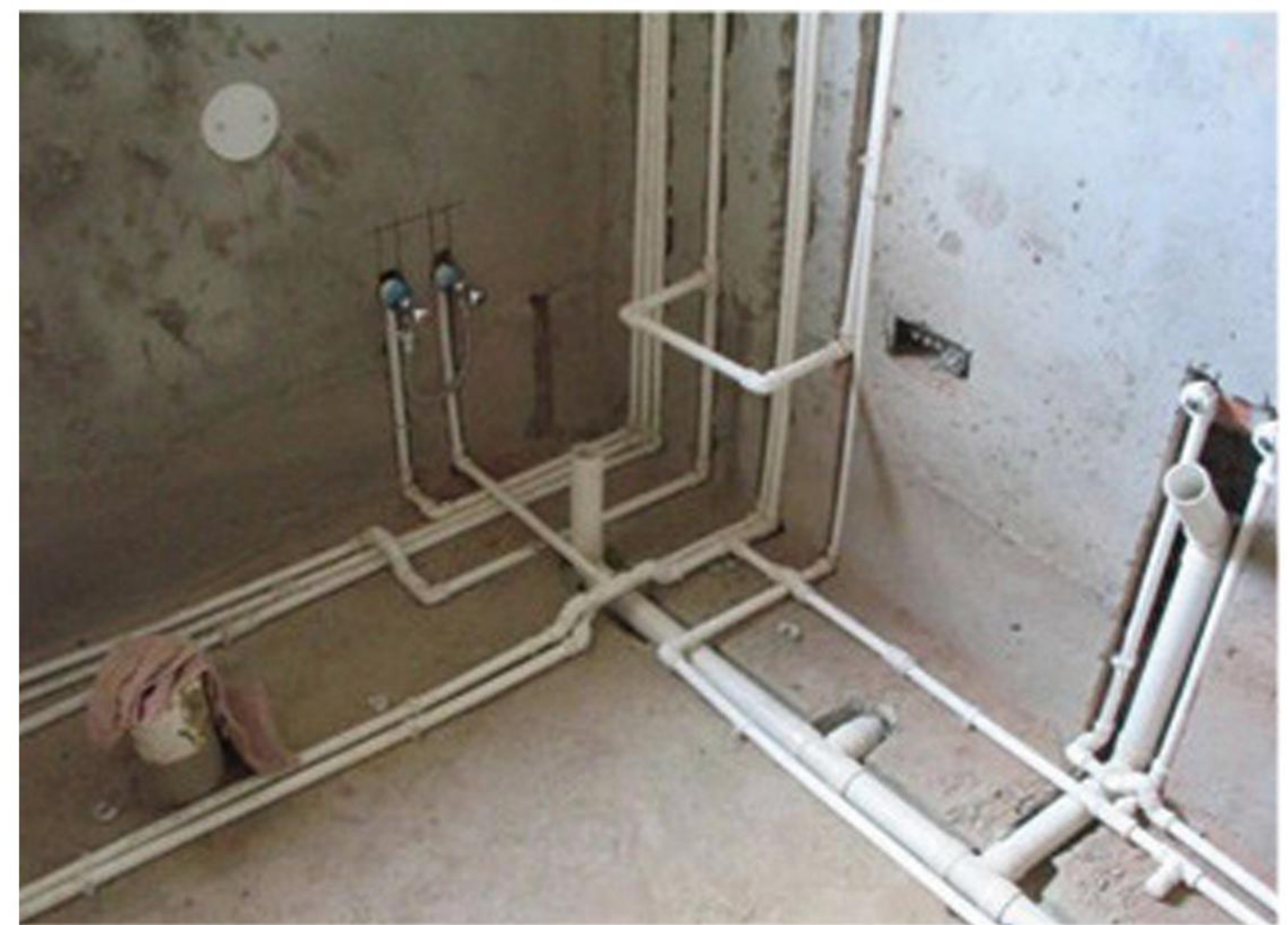
Hydropower engineering installation
