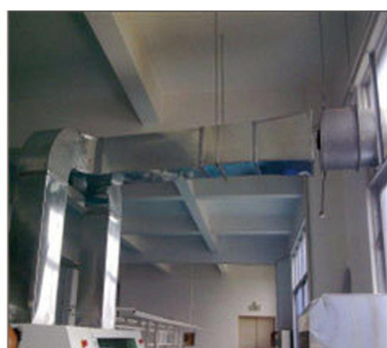
Exhaust pipe installation
