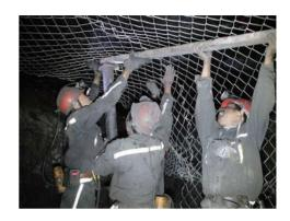
Diamond mesh is the earliest steel wire mesh for coal mine supporting mesh. It is widely used as the artificial support, tunnel support and side support. The diamond mesh can also cover the mine to prevent minerals and other stones from falling down as mine security fence.
